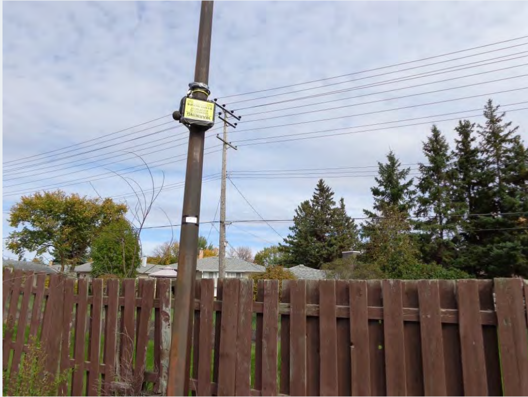
Photo 5: Monitoring Point 5 – Versatile Storage (facing northeast)
