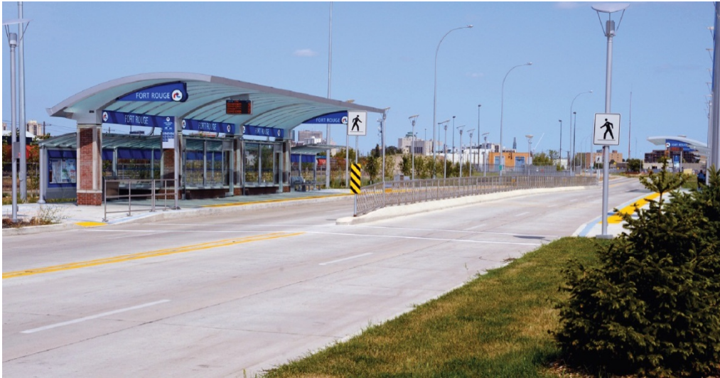
Figure 3: Illustrative Photo of Station Design (existing Fort Rouge Station)
